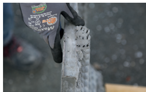
© Baustädter – TU Graz
