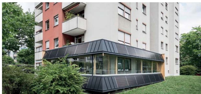
Figure 3: The thermal shell: a steel-wooden shell with glass and photovoltaic elements was installed on the surface of the building, which drastically lowered the energy demand.
