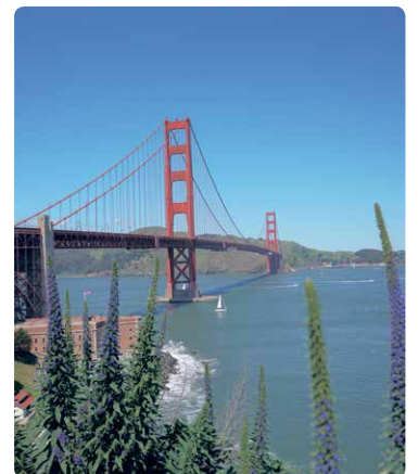
Golden Gate Bridge.
