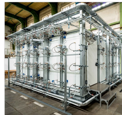
CLIMATE ROOM part of the Combined Energy Lab. 2.0
