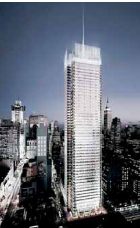
New York Times, New York City/USA Architekten: Renzo Piano Building Workshop, Genua/I New York Times, New York City/USA Architects: Renzo Piano Building Workshop, Genoa/I
