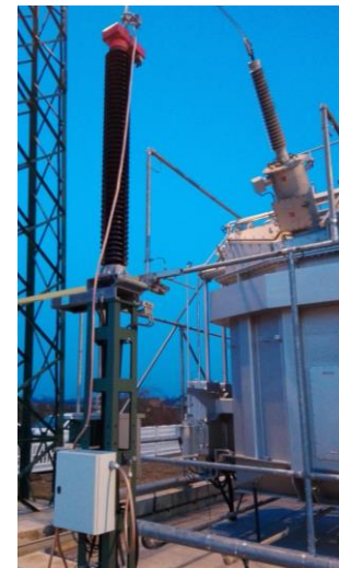
Fig. 2: Transformer Neutral Measurement
