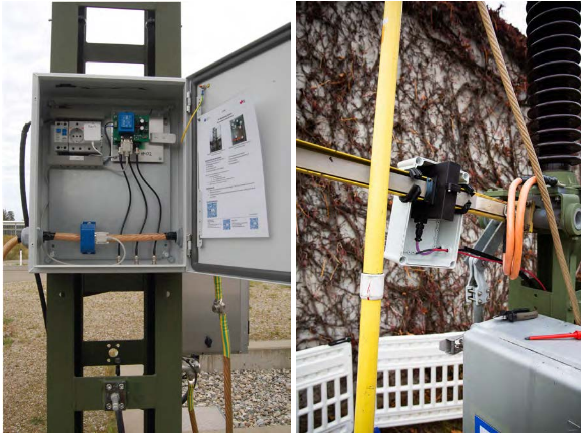
(a) Installed transformer neutral point current measurement system with open cabinet.
