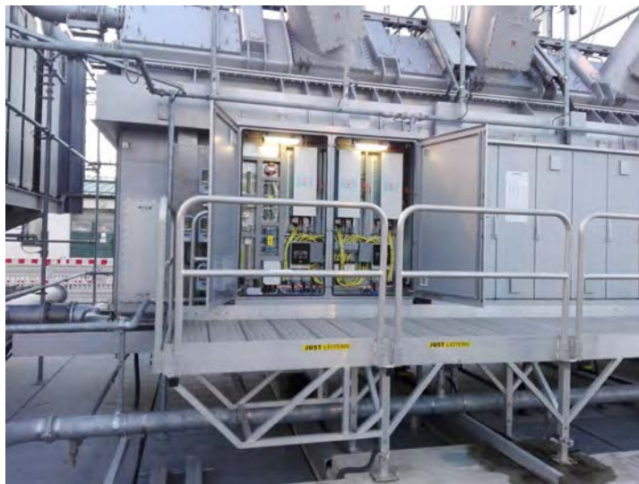
Figure 2.31: DCC cabinet at 400/110/30 kV 300 MVA transformer.
