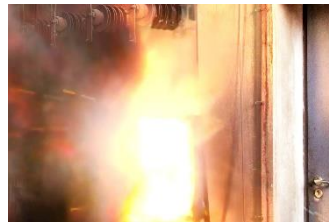
High Power DC Testing
