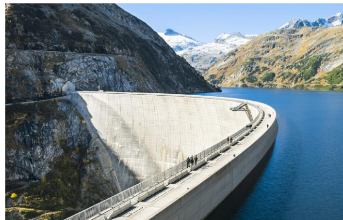
© Pökl F.G., ATCOLD 2018 Pumped Storage Hydropower in Austria
