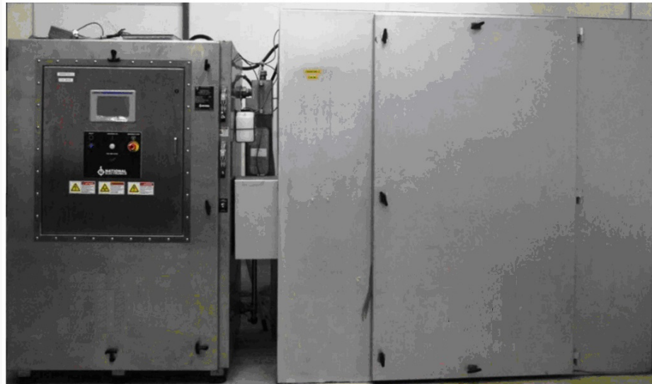
Fig.7 Pilot microwave heating system used for experimental program
