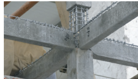
Construction of the precast RAC frame
