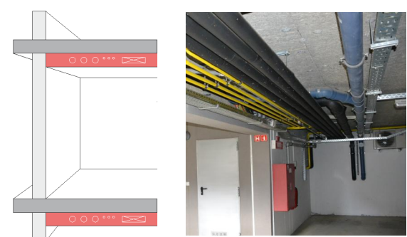
Cable arrangement below horizontal building components
