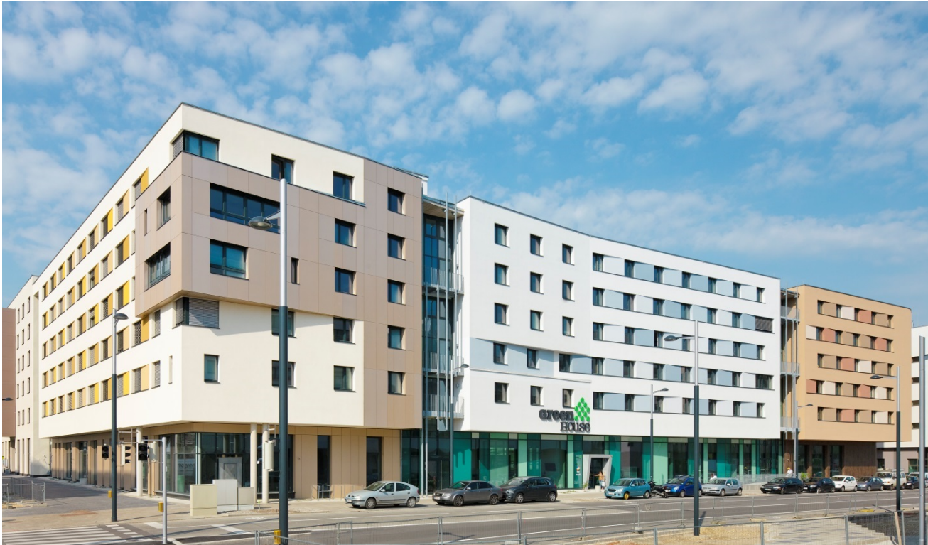
Austria's first „Passive House Plus“ student dormitory in Vienna
