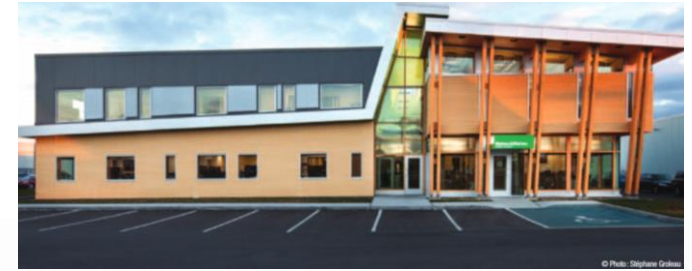
Maheu&Maheu's head office, first wooden load-bearing glass wall, Qc (Cecobois)
