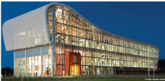
GlaxoSmithKlined's office building, Qc (Cecobois)
