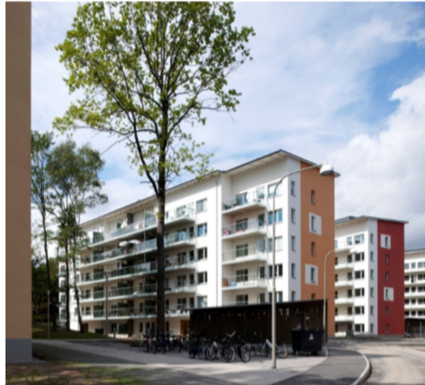
Image: Blå Jungfrun energy efficient apartment project in Stockholm, 2010 (Source: 4)
