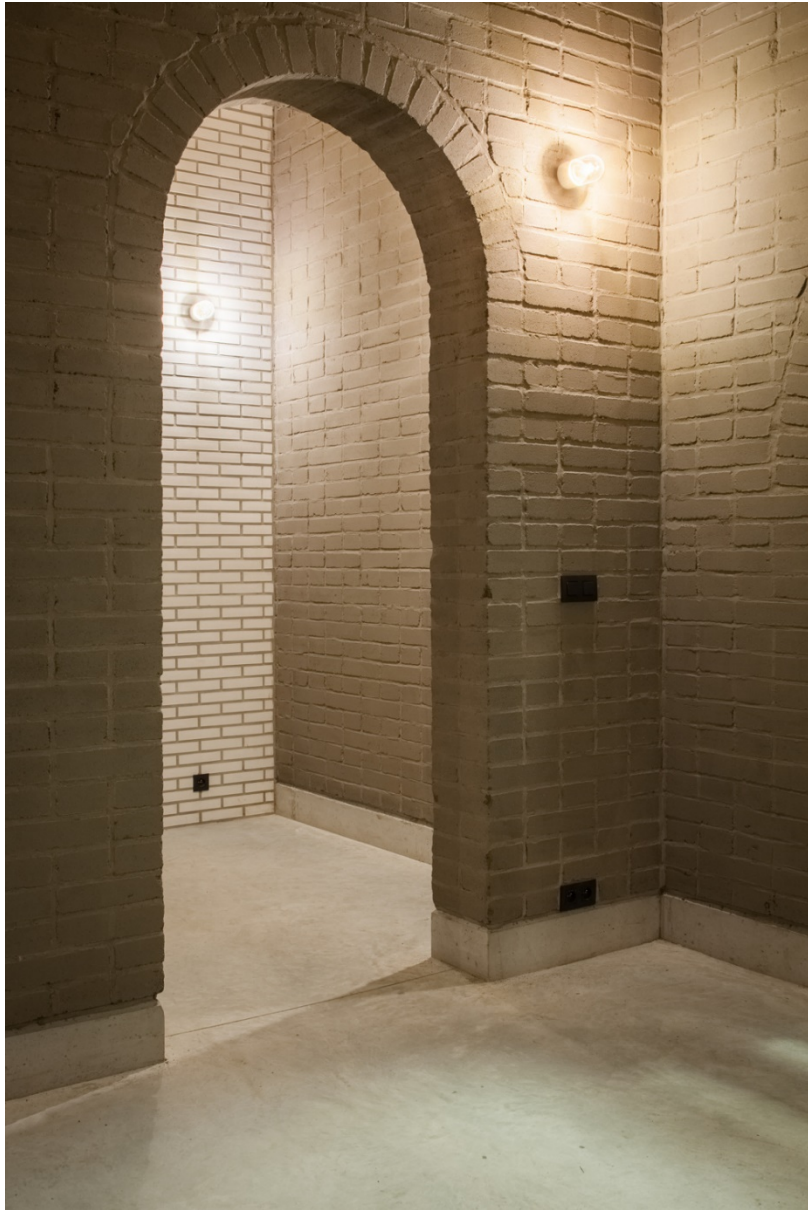
Bioclass, Edegem, 2018 Load-bearing compressed earth bricks (Thomas Noceto)
