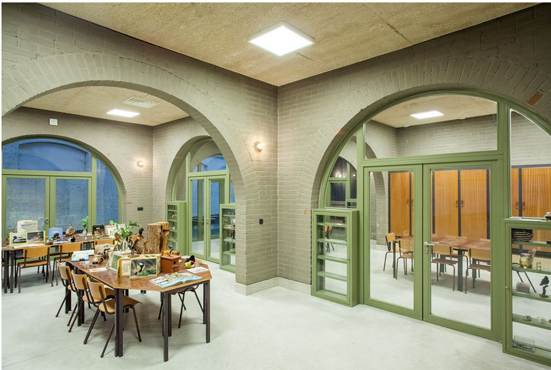
Bioclass, Edegem, 2018 Load-bearing compressed earth bricks (Thomas Noceto)
