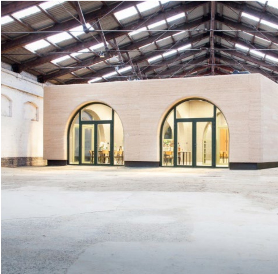
Bioclass Edegem (Antwerp), 2018 Load-bearing compressed earth bricks (Thomas Noceto)
