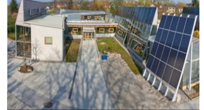
new constructed office building
