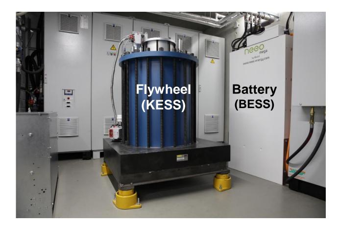
The system is integrated into a model factory aiming to increase its flexibility
