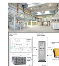
Smart Electricity Systems and Technologies Laboratory (SmartEST) AIT Austrian Institute of Technology, Wien
