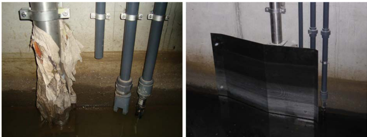
Figure 1-5: Probe clogging with hygiene products (left), installed sheet metal cover prototype (right) (Images: Graz University of Technology, 2014)
