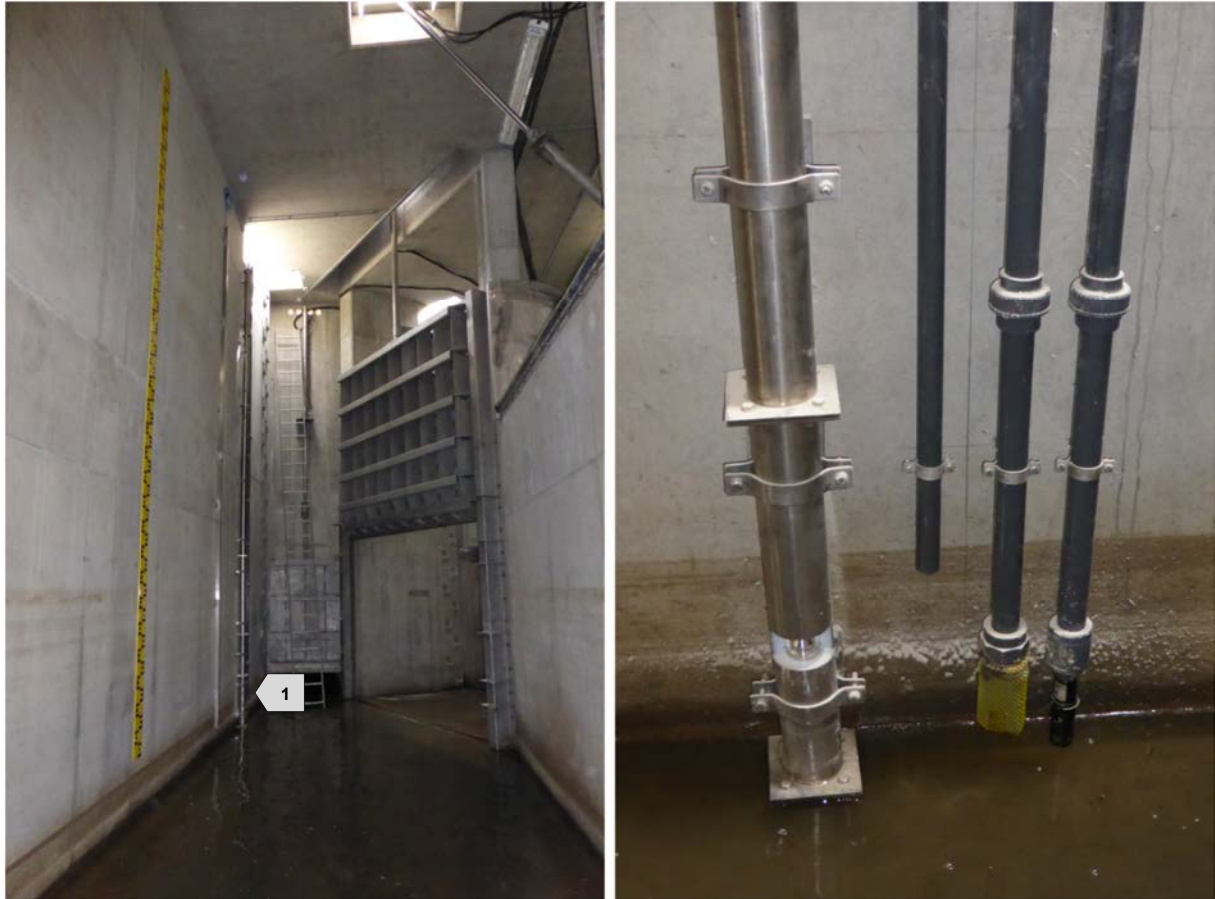
Figure 1-3: Probe installation at Graz-CST-CS1 in control structure CS 1 (left, [1]) and front view of the probes (right) (Images: Graz University of Technology, 2014)
