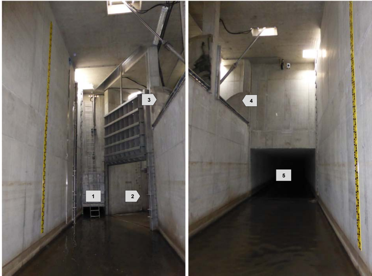
Figure 1-2: Sluice gates to WWTP Graz [1] and to the river Mur via the overflow channel [2] and moveable weirs to the overflow channel [3], [4]; storage volume upstream of CS 1 [5] (Photos: Graz University of Technology, 2014)
