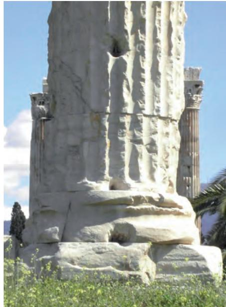
Fig. 6.2: Relative displacement between two drums close to the base of a column of the Olympieion.
