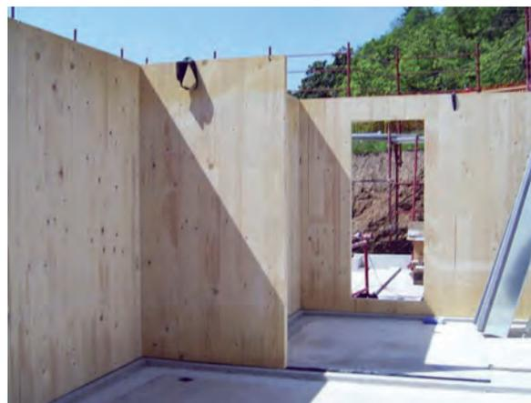
Fig. 3.2: X-lam walls in a building (copyright IVALSA-CNR)
