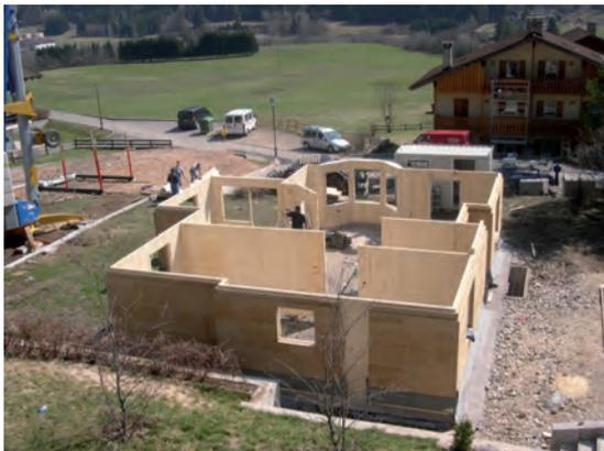
Fig. 3.1: Typical X-lam building (Photo Rasom wood technology)
