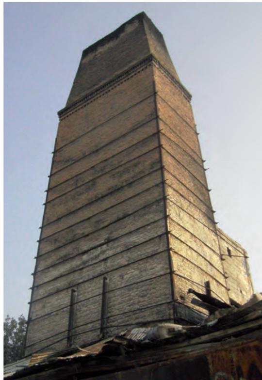
*Fig. 7.4: Masonry chimney confined by metal hoops.*
