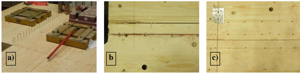
Figure 2.16: Screw connection of CLT elements in plane: a) drilling; b) single row; c) additional screw rows for reinforcement against tensions perp. to grain
