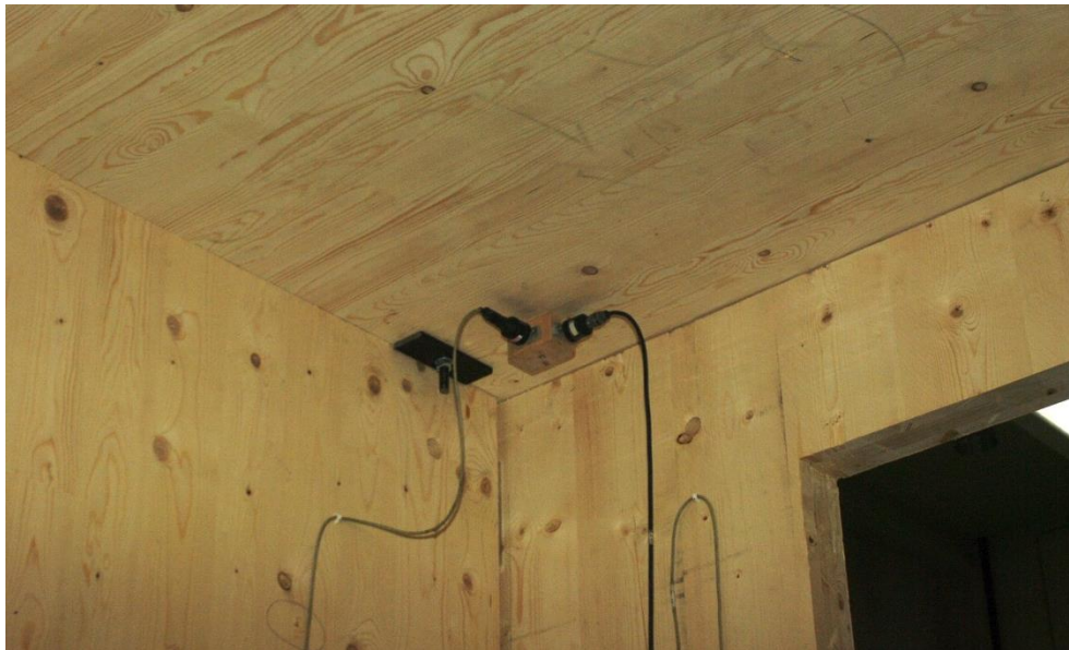
Figure 3.5: Detail of the accelerometers placed inside the building
