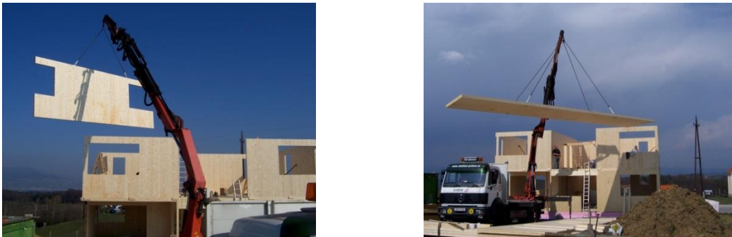
Figure 2.2: Use of CLT for a single family house [source: holz.bau forschungs gmbh]
