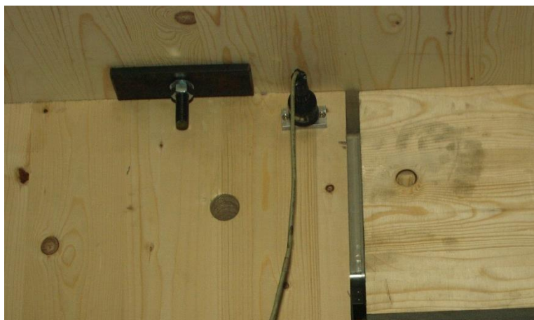
Figure 3.6: Detail of the accelerometers placed on the wall
