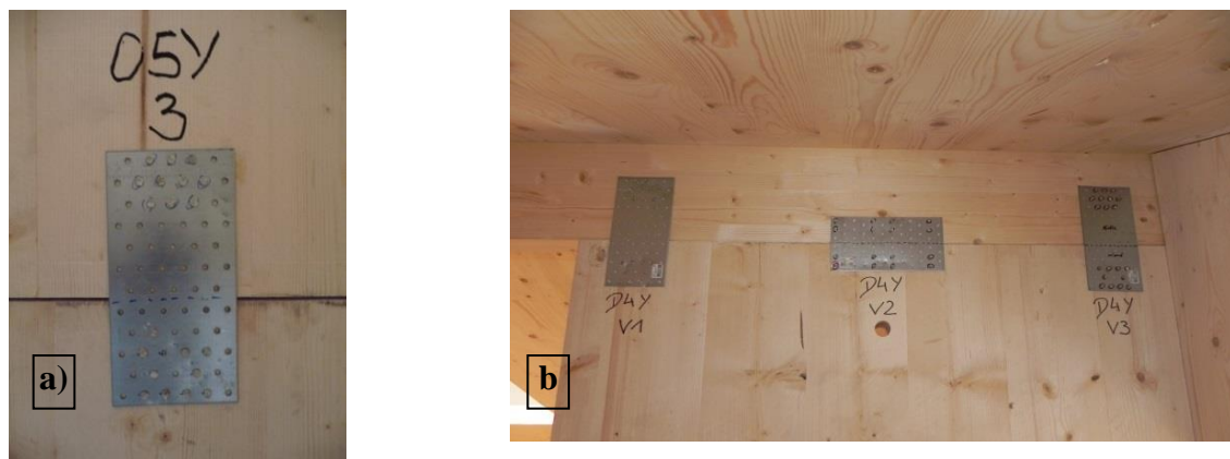
Figure 2.14: Nail plates: a) wall – wall; b) ridge purlin – wall
