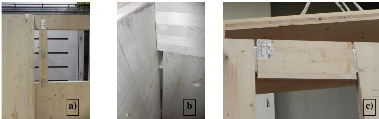
Figure 2.18: SHERPA(R) connector: a) assembling; b) wall - wall joint; c) lintel joint
