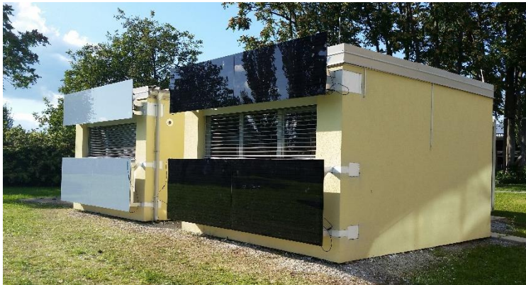
Test building with autonomous cooling PV system
