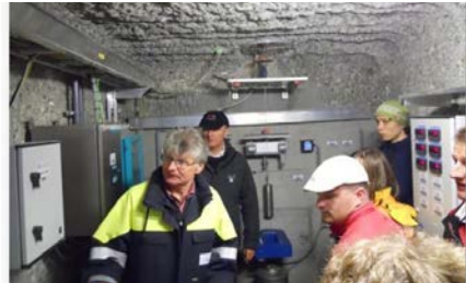
Lotkammer - KW Salza | Monitoring chamber - HPP Salza
