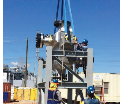
Figure 8: Aftercooler being lowered into position (Courtesy: Heatric)
