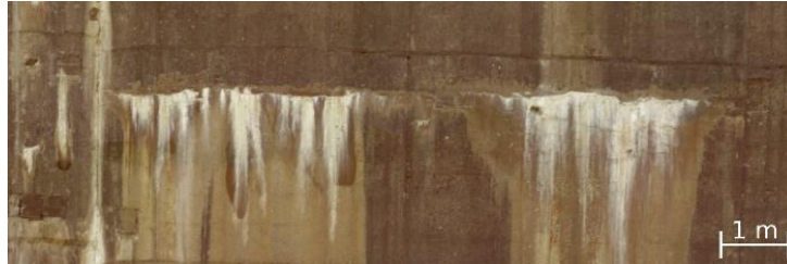
Figure 6: Orthoimage of a defect region on the downstream side of the Drossen dam (block 16), derived from 21 OAC textures (1 pixel corresponds to 2 mm on the surface)
