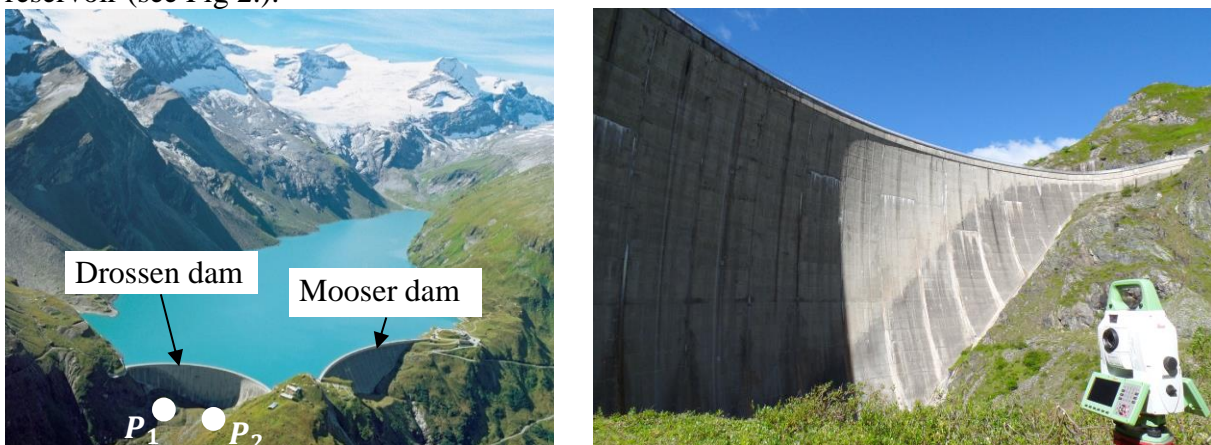
Figure 2: Measurement site, overview image showing the two concrete dams of the reservoir Mooserboden (left, source: Verbund), frontal view on the downstream side of the Drossen dam with the instrument set up at point P_1 (right)
