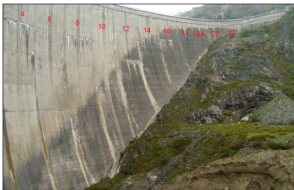
Figure 1: Photograph of the downstream side of the Drossen dam (left), corresponding CAD drawing showing defect locations (right, Verbund, 2011)
