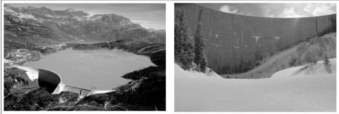
Fig. 1. Overview of the hydroelectric power dam Kops (left) [1] and the vertically aligned concrete blocks of the arch dam, each about 30m wide (right)
