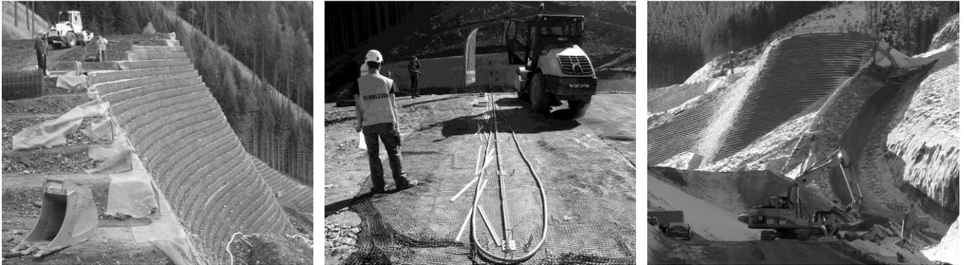
Figure 1. Reinforced earth structures at Longsgraben, Access ramp (left), installation of fiber optic sensing cable on the geogrid (center) and steep slope section (right)
