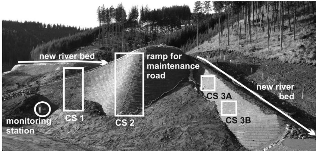
Figure 3. Overview of the cross sections of the reinforced earth structures
