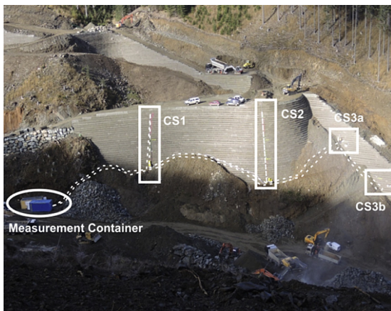
Fig. 13. Monitored cross sections at the Longsgraben disposal site.
