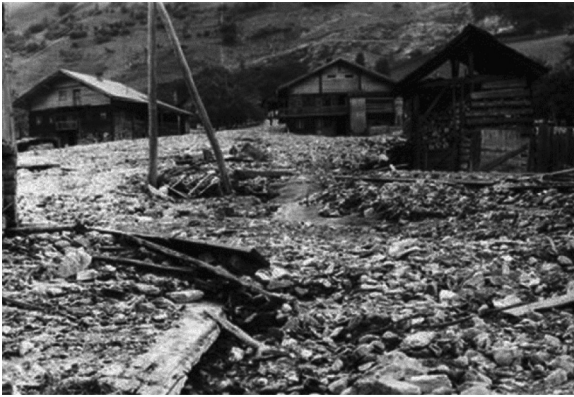
Fig. 1. Damages in the village Doellach in Austria as a consequence of the Gradenbach landslide.
