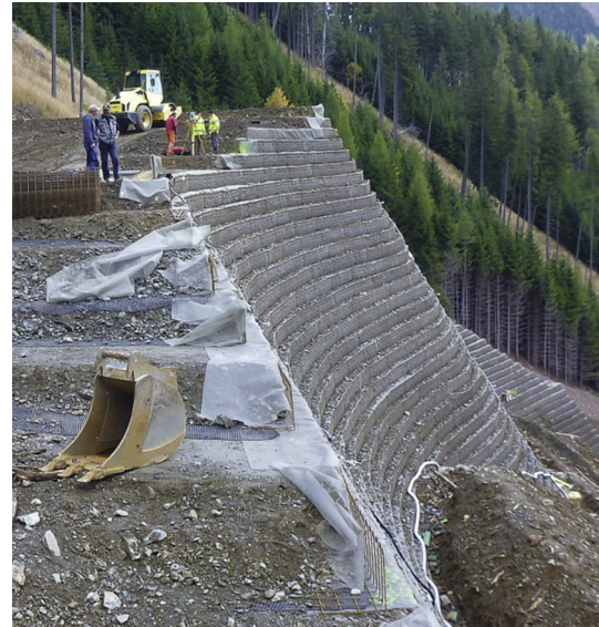
Fig. 11. Construction of the reinforced earth ramp of the maintenance road.
