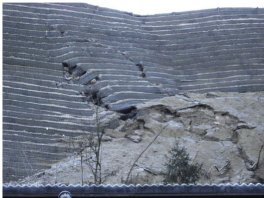
Fig. 2. Failure of reinforced earth structure at the road B320, Austria (Liezen Online, 2011).
