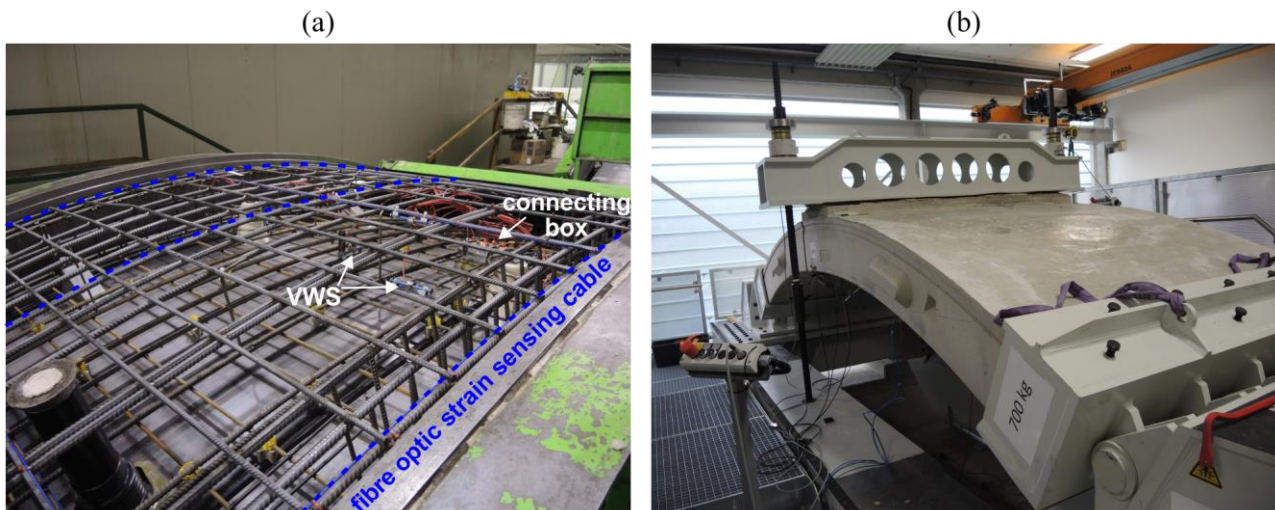
Fig. 4: (a) Installation of the fibre optic sensing cable along the reinforcement bars and (b) test rig for precast tunnel lining segments
