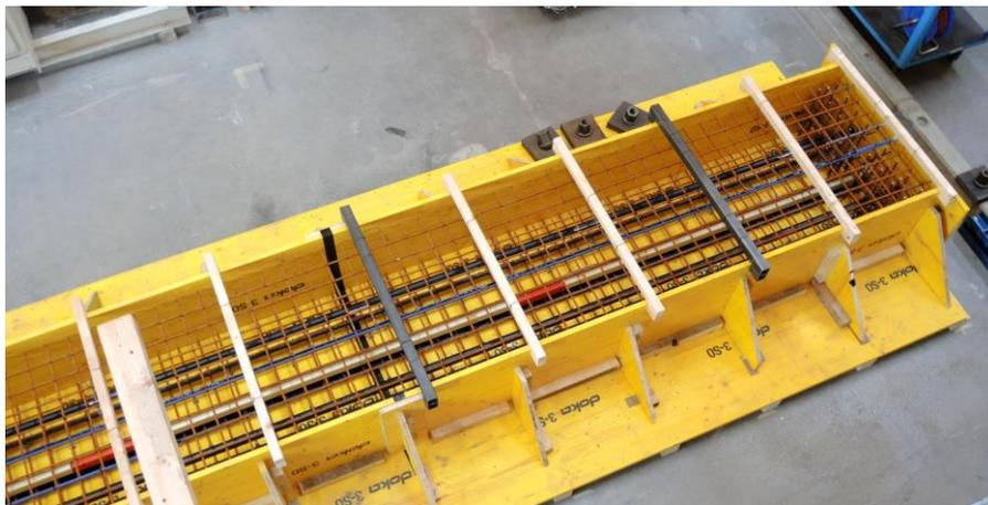
**Figure 2. Production of concrete beam structure**
