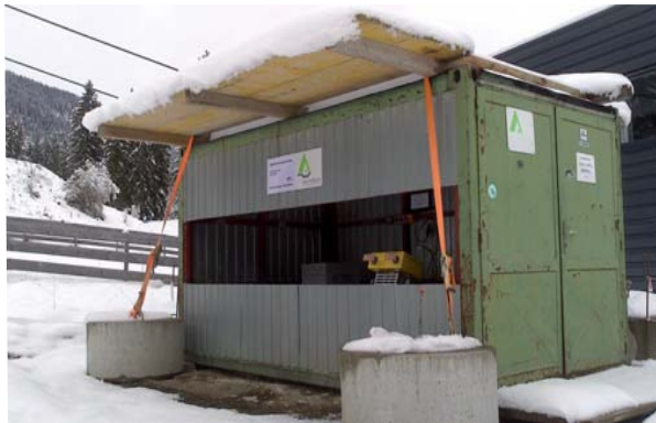
InSAR deployment in Reutte, Tyrol for the remote (2.2 km) measurement of rock wall deformation.
