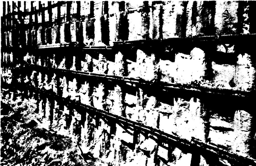
Figure A-2 — Drilled concrete shafts supported by three levels of tie-backs and walers.
