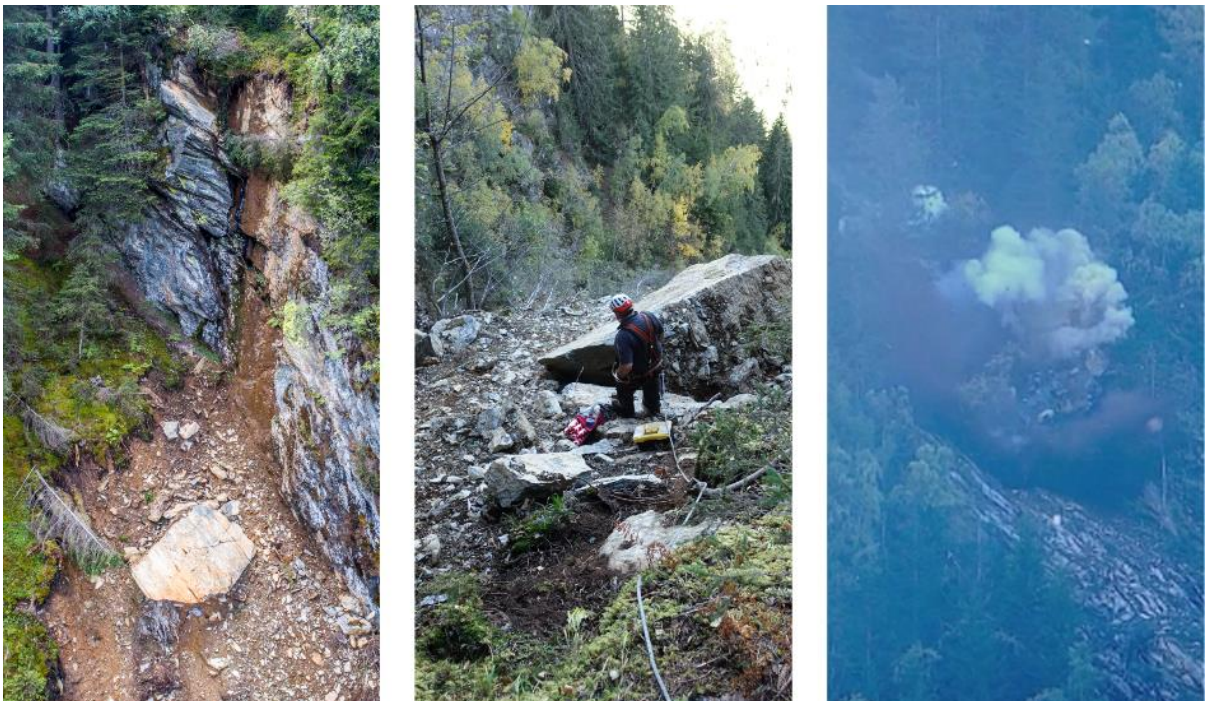
Figure: Rock fall hazard close to the Ursprungalm in the alpine region of the municipality of Schladming. Left: Photograph taken from helicopter on August 9th, 2021; Centre: Installation of the blasting charge by experts on October 18th, 2021; Right: Photograph of the explosion taken from the opposite side of the valley. Copyright: Rainer Kienreich (Graz University of Technology, Institute of Rock Mechanics and Tunnelling)
