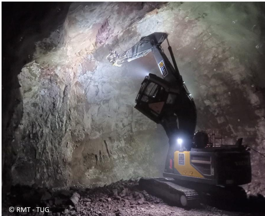
Figure: Blasting lengths of up to several meters require special equipment for scaling works.
