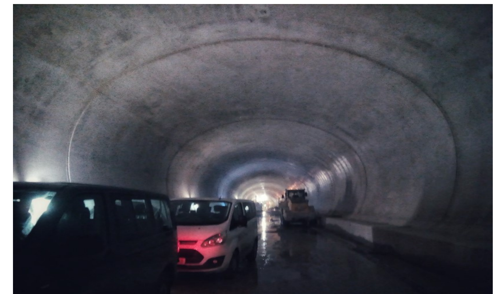
Fig. 11: FINAL LINING LAYER IN THE BBT TUNNEL.
