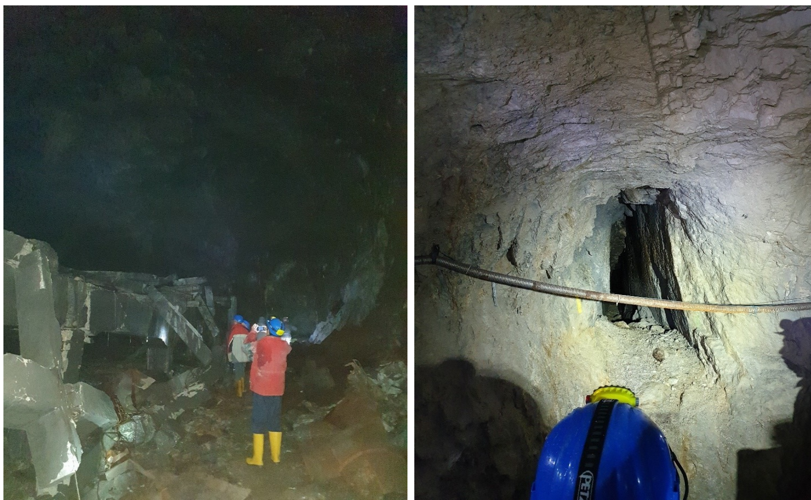
Fig. 3: LEFT: ONE OF THE BIGGEST CAVERNS IN THE SYSTEM. RIGHT: TUNNEL FOLLOWING DISCONTINUITY.
