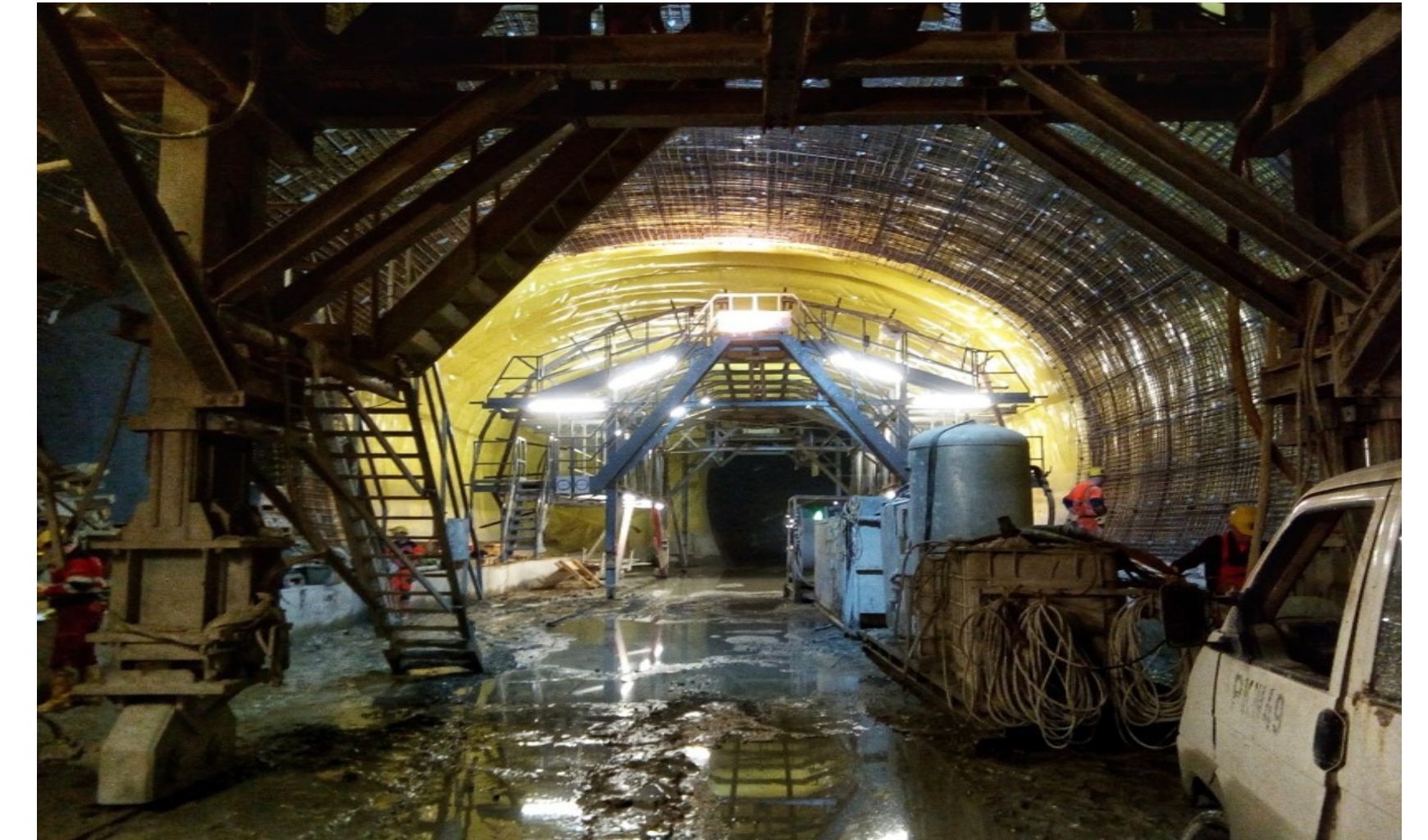
Fig. 9: FORMWORK STAGE FOR BBT TUNNEL FINAL LINING.
