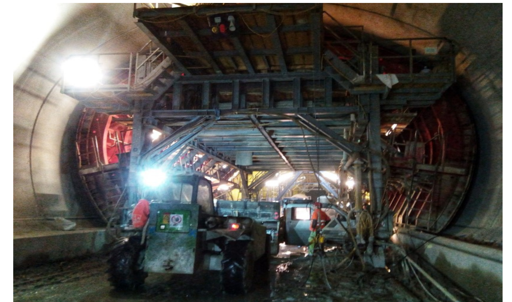
Fig. 10: FINAL LINING CURING STAGE FOR BBT TUNNEL.
