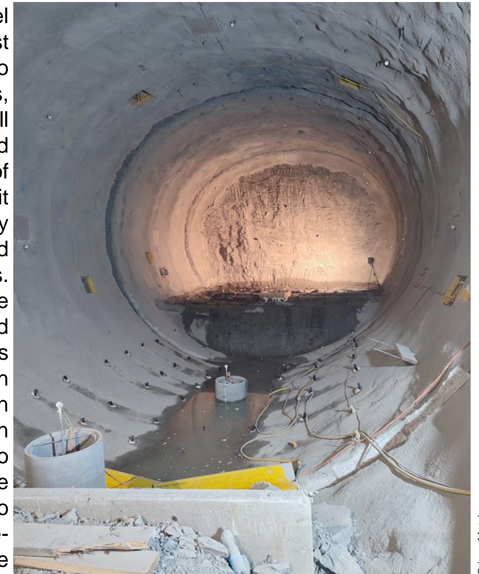
Test gallery in cross-passage of the Angath adit tunnel.
