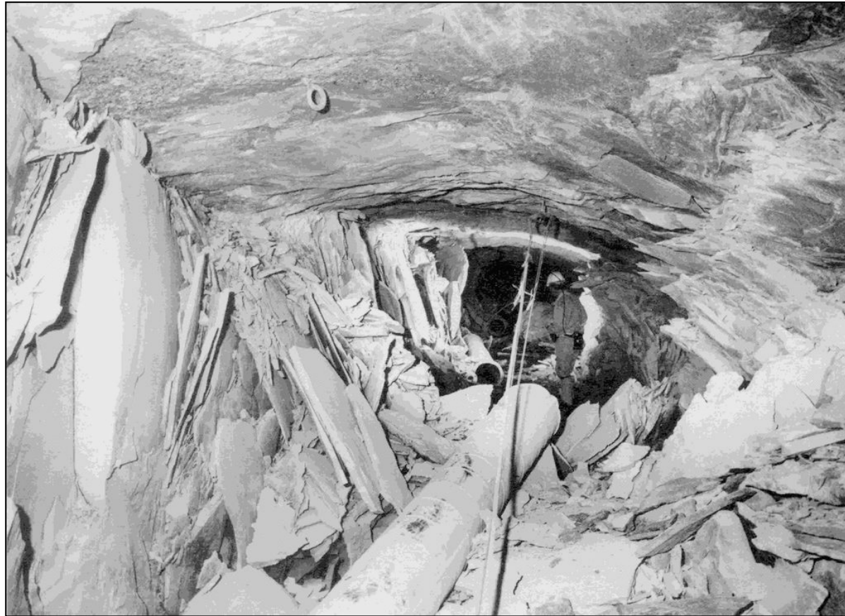
Rockburst - Example of brittle failure in mining and tunnelling (Ortlepp, 1997)
