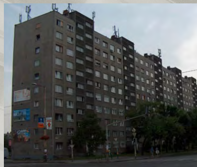
Terraced panel building with narrow strip blocks
