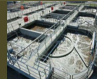
Two-stage plant with anaerobic digestion in Kirchbichl (AT)
