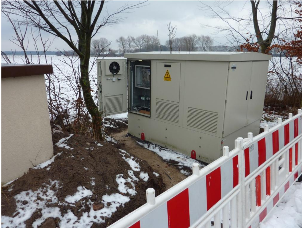
SGB- Kompaktstation in Vissel
