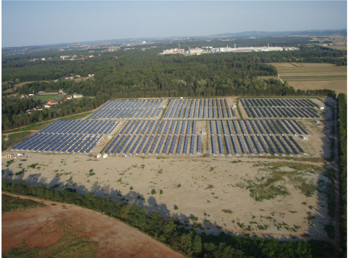
Solar field near Kidričevo (biggest in Slovenia) installed 6MWp on cca. 11 ha area
